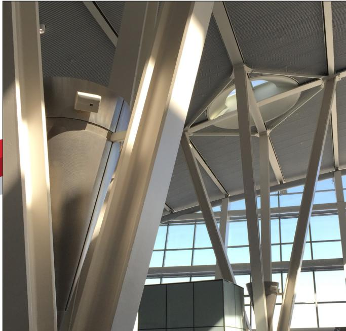
**Firefilm IV** cures to a very smooth, decorative finish so no topcoat is required. It features fast cure times for improved production of up to two coats per day. Firefilm IV is LEED-compliant and features extremely low VOCs at 4 g/l.
