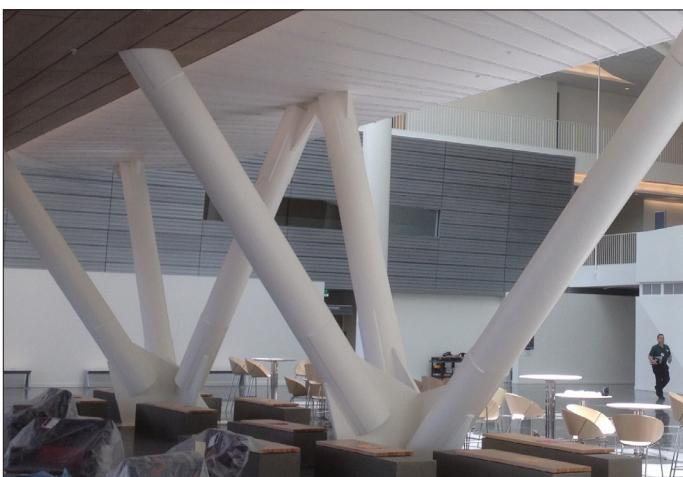
**Firefilm III** cures to form a smooth to slight orange peel finish that is durable and resistant to impact and abrasion. It is widely compatible with topcoat options, is LEED-compliant, and features very low VOCs at 20 g/l.
