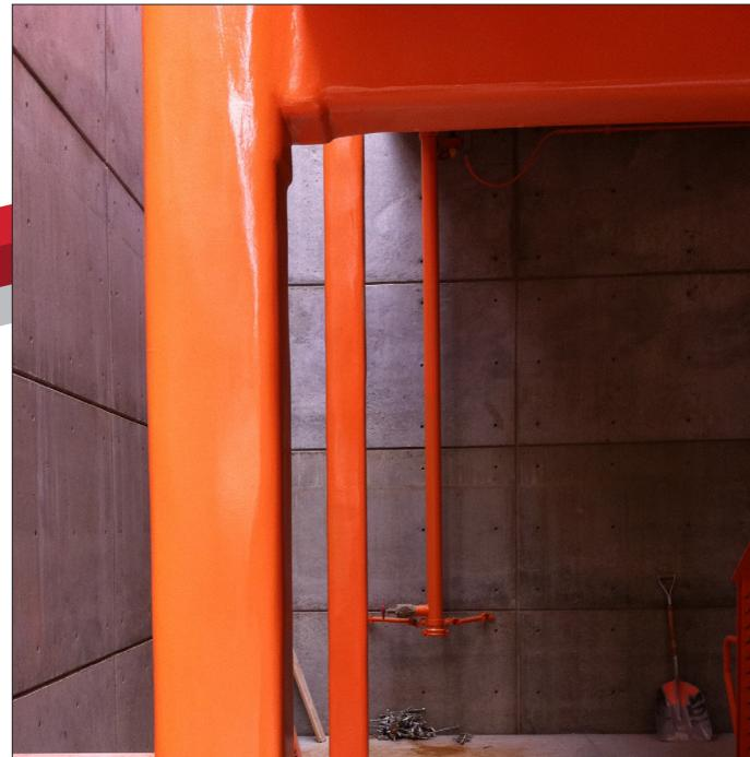
**Thermo-Lag E100 S** is a 95% solids epoxy intumescent coating with similar performance to Thermo-Lag E100 but formulated for single-component application. Single-component application involves less complex equipment requirements and is preferred for field installation. Very low VOCs at 64 g/l.
